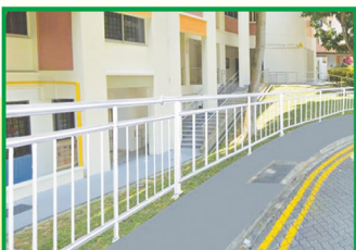
Widen Footpath - Blk 267 to 268, Blk 278 to 287
