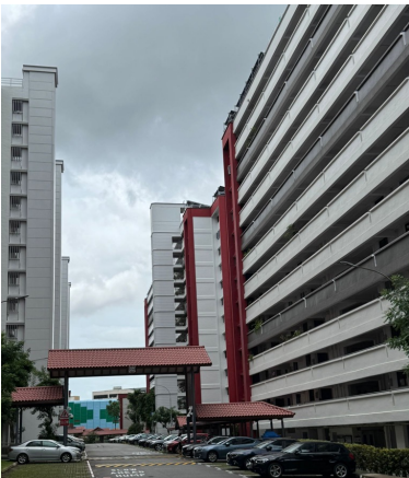
Repairs & Redecoration @Shunfu
