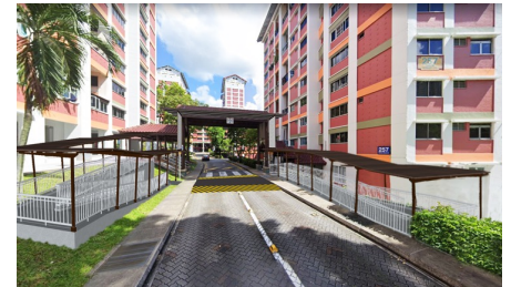
New Covered BFA Ramp Access at Blk 261 & 257 (2Q 2025)
