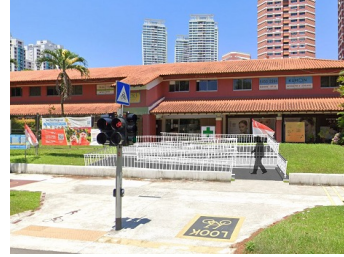
New Open BFA Ramp at Blk 283 (2Q 2025)
