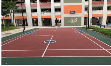
Upgrading of Existing Badminton Court at Blk 266 & 268 Bishan St 24 (Completed)
