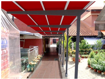
New Covered Linkway between Blk 279 & 280 (Completed)
