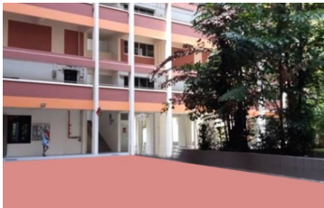
Upgrading of Open Space Flooring at Blk 261 (2Q 2025)
