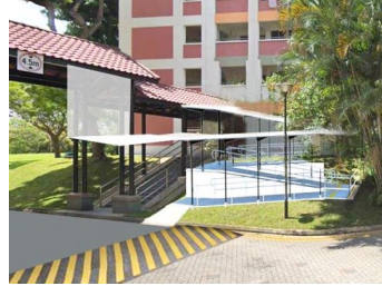
New Covered BFA Ramp from Blk 263 to 264 (3Q 2025)
