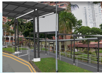
New Drop-Off Point with Covered BFA Ramp at Blk 285 (2Q 2025)
